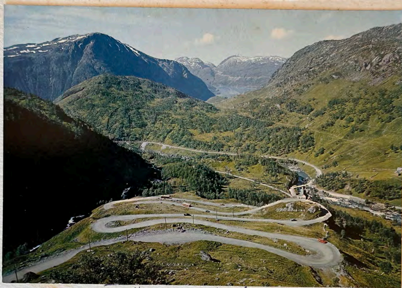
Roldal. The Custmannli hairpin bends on the Hardanger Telemark Rd.
